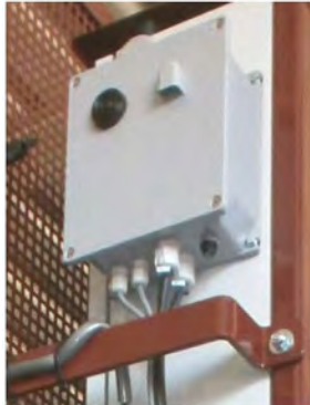
Example of installation of a panel
